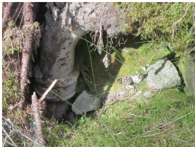
but all that remains now is a stone and this water pipe.
