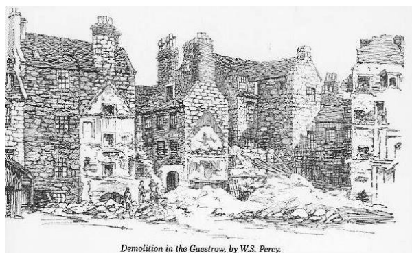
Demolition in the Guestrow, by W.S. Percy.
